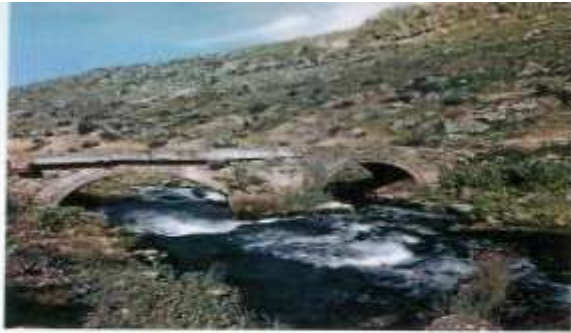
Two-arch bridge, Minkarid village
