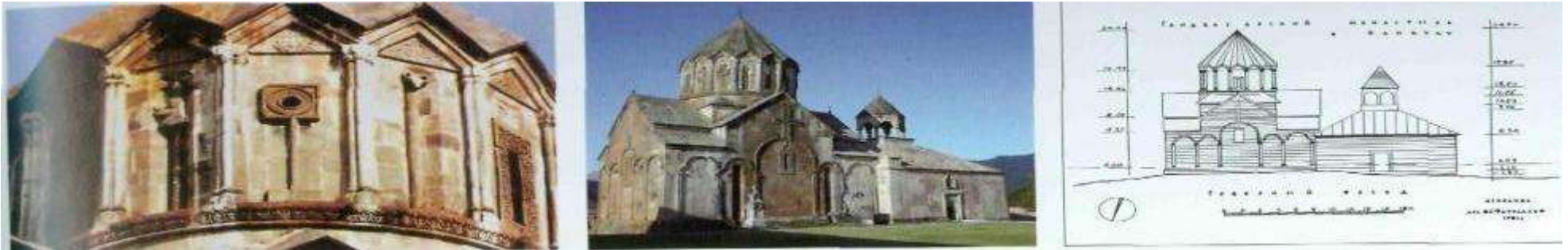
Photos and scheme Ganjasar cloister, Vangli village
