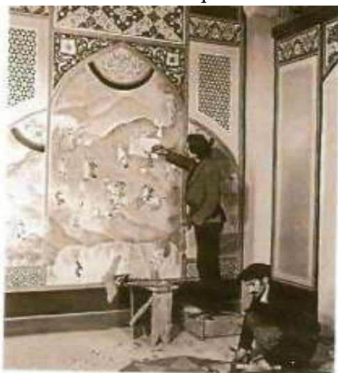
Restoration works in Saatly mosque
